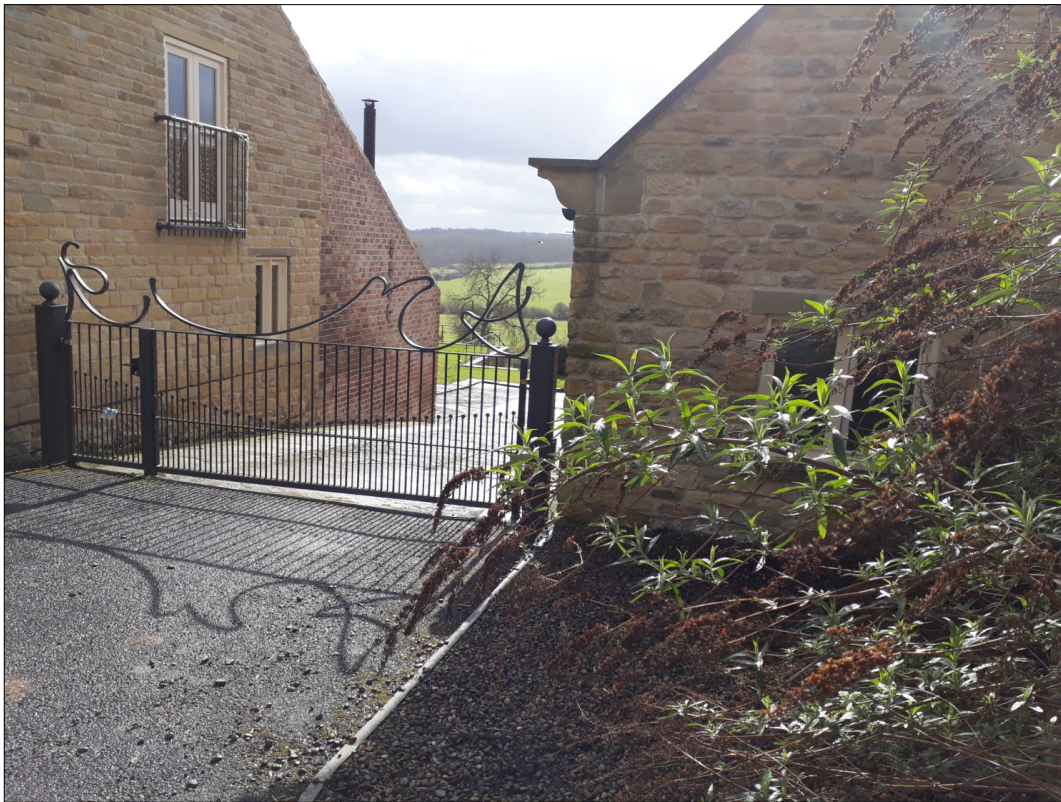
'Important view' through Hall House Farm. The application site is sited further to the left than the viewpoint allows a visitor to see
